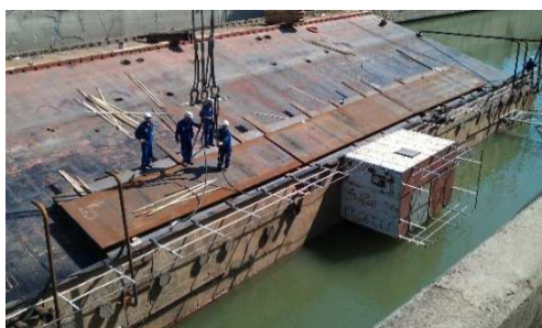
Fig. 26 Placing additional steel plates to get the sealing gasket zone out of water
