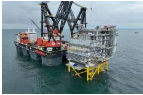
Figure 1 EA3 HVDC topside lifted into place [1]
