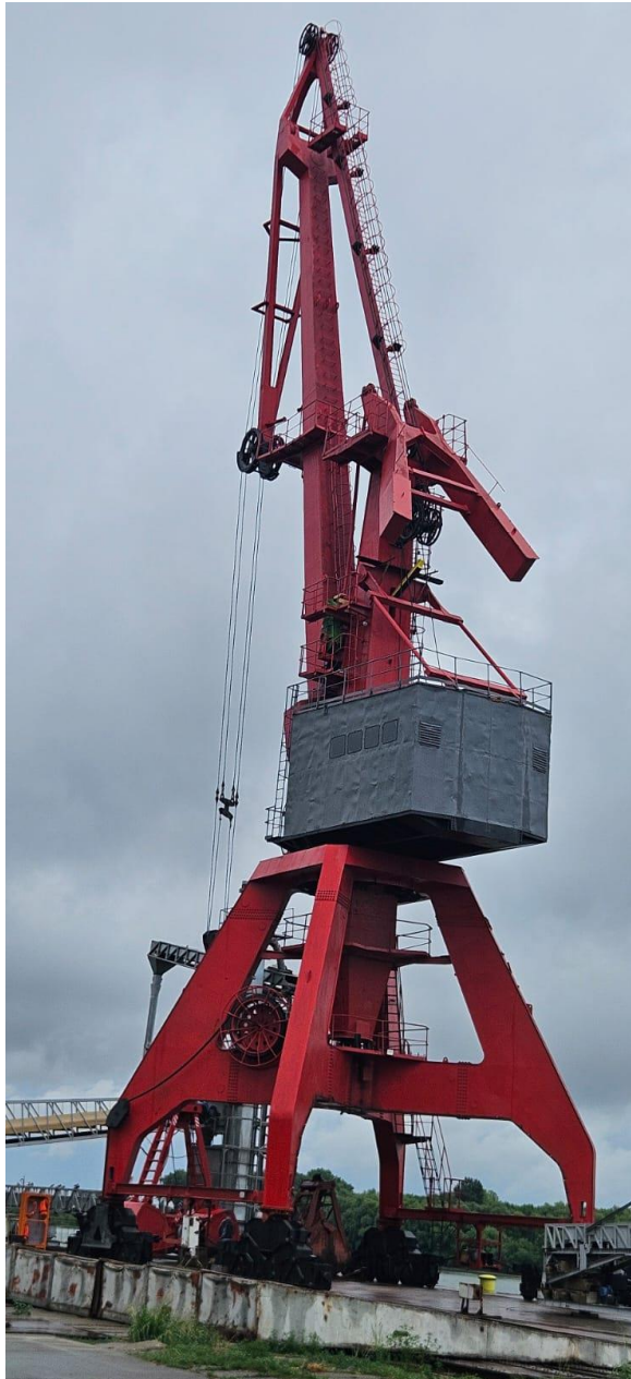
Figure 1 Rail-Mounted Portal Slewing Crane
