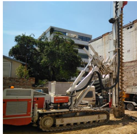
Figure 2 Micropiles drilling rig
