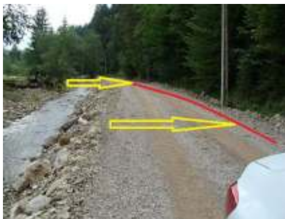
Fig. 5. General view of the Voroneţ River shore erosion at the limit of the road DJ 177D in the downstream area after the flood of June 2016 (photo Aug. 2016 [4])
