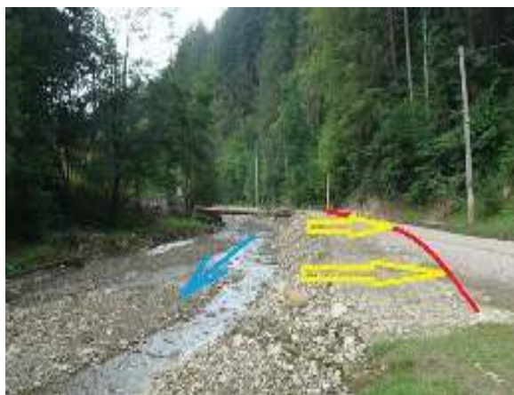
Fig. 6. Details of the Voroneţ River's erosive action on the left bank and the road DJ 177D: a - the beginning of the deforestation degradation and the erosion of the road (downstream "Camp Cristea"); b - the end zone of the eroded road section to the slope (upstream of the Brusturosu Brook) [4]
