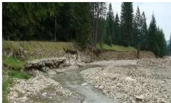
Fig. 5. General view of the Voroneţ River shore erosion at the limit of the road DJ 177D in the downstream area after the flood of June 2016 (photo Aug. 2016 [4])
