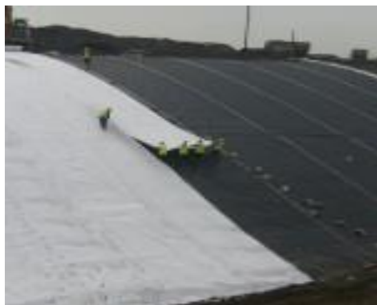
Fig. 5. Protection from geogrid + geotextile mounted on the profiled river bank [9]
