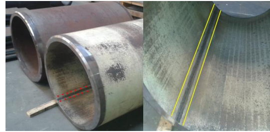
Fig. 16. Completion of the welding operation
