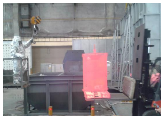
Fig. 23. Introduction of the cylindrical bed frame elements in the basin with bubbling water
