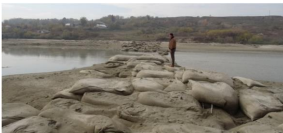
Fig. 12. General view of the structural degradation of a bottom threshold made from geo-bags under hydrodynamic action (photo, Sion, 2019)
